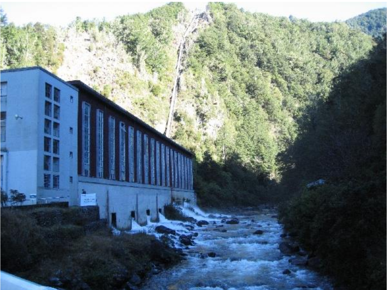
Figure 3-7: Cobb Power Station (taken from trustpower.co.nz ).
